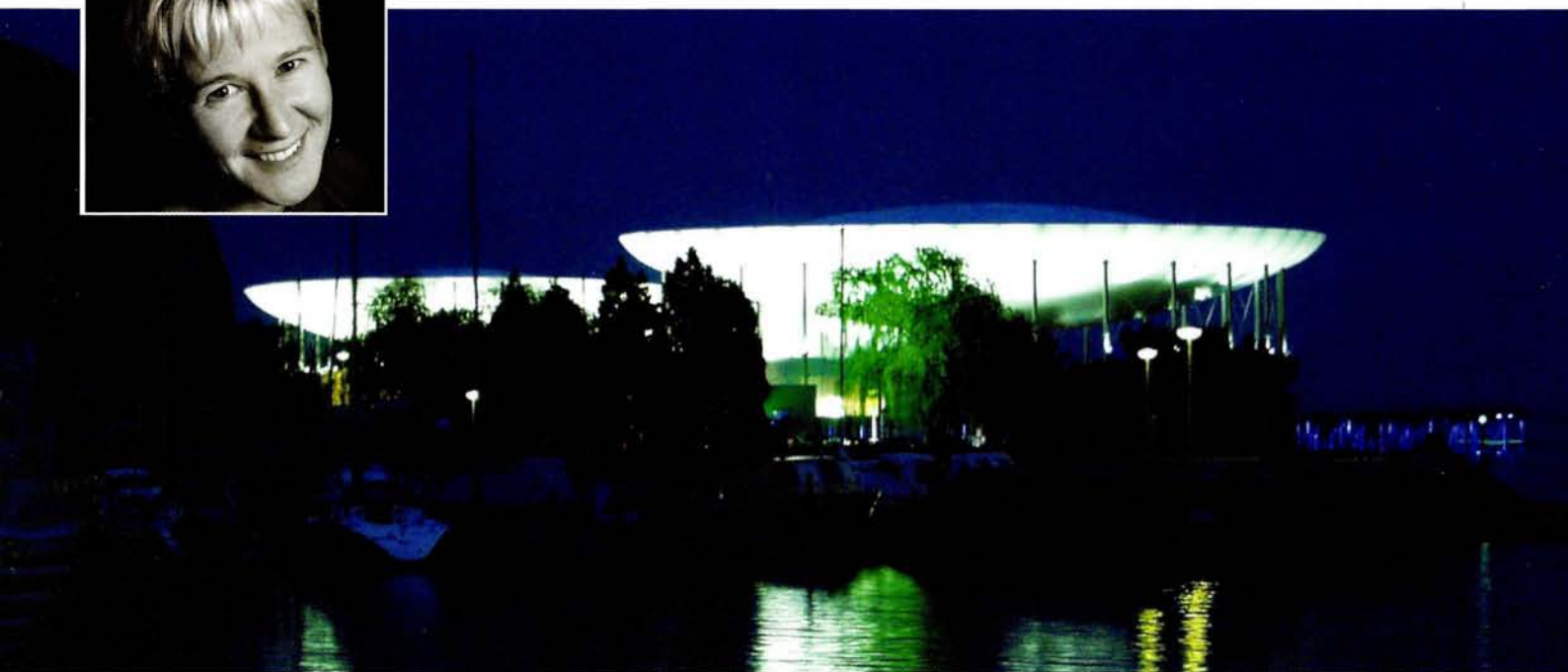
Power and telecommunication cables / Neuchâtel Arteplage
