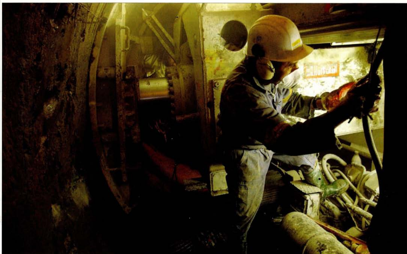
A tunnelling machine digs the last few metres of the decay tunnel for the CERN neutrinos to Gran Sasso beamline in May.
